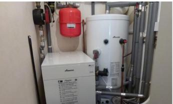
A new boiler, hot water tank and all of the associated plumbing, including a separate oil tank outside provides a separate system for the Village Hall.
